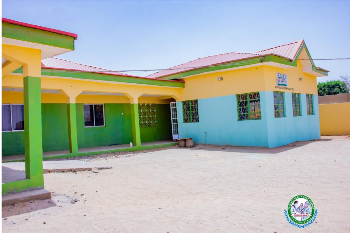
KATSINA ZONE PHC DUTSIN-MA LGA
